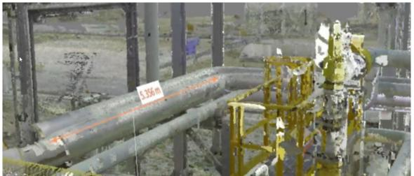
Figure 1. Measuring distance between inaccessible points using augmented reality and 3D photorealistic model.
