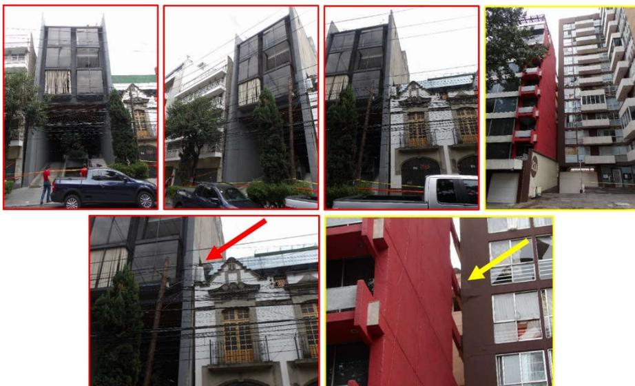
**Figure 16:** Damage induced by pounding between closely spaced buildings due to the September 19, 2017 earthquake (from Lekkas et al. 2017).
