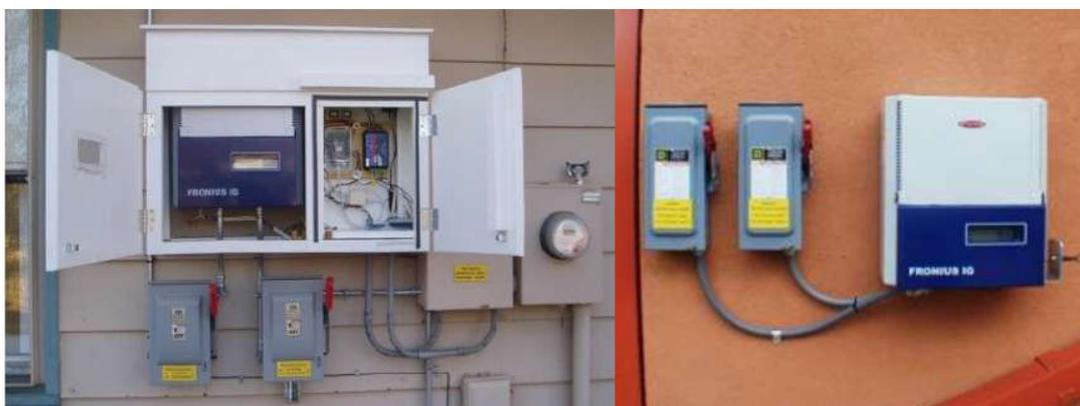
Figure 3: Inverters with their disconnect switches used in PV units (Hellenic Fire Brigade 2015)
