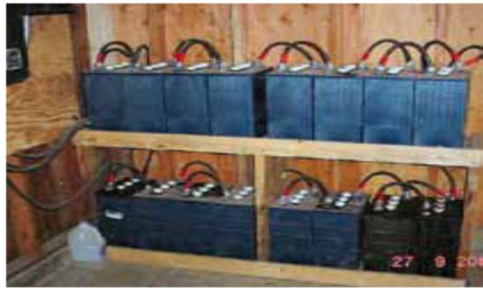
Figure 5: Batteries of a standalone PV system (CAL FIRE 2010)
