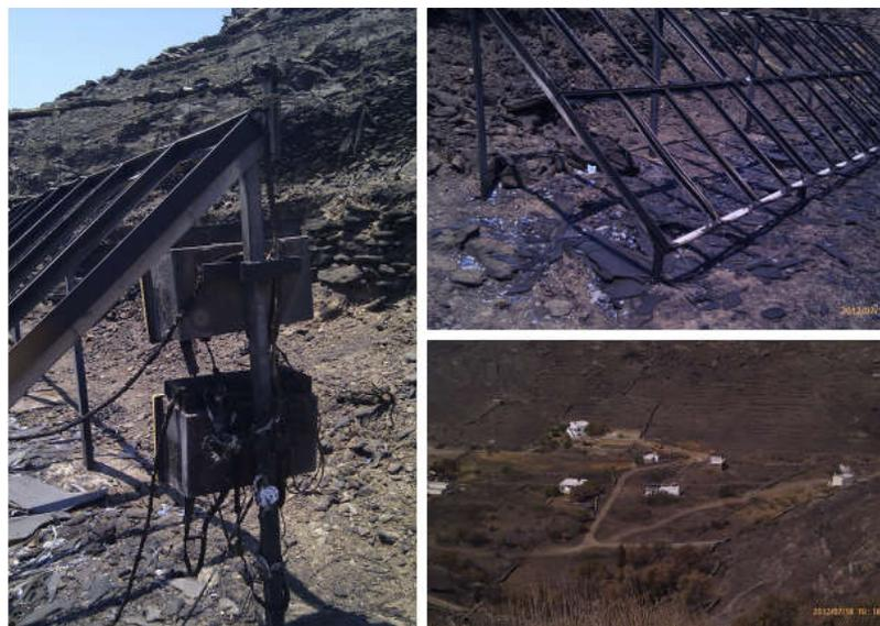
Figure 12. Forest fire spread into a PV unit in Kythnos, Greece in 2012 (Hellenic Fire Brigade 2015)
