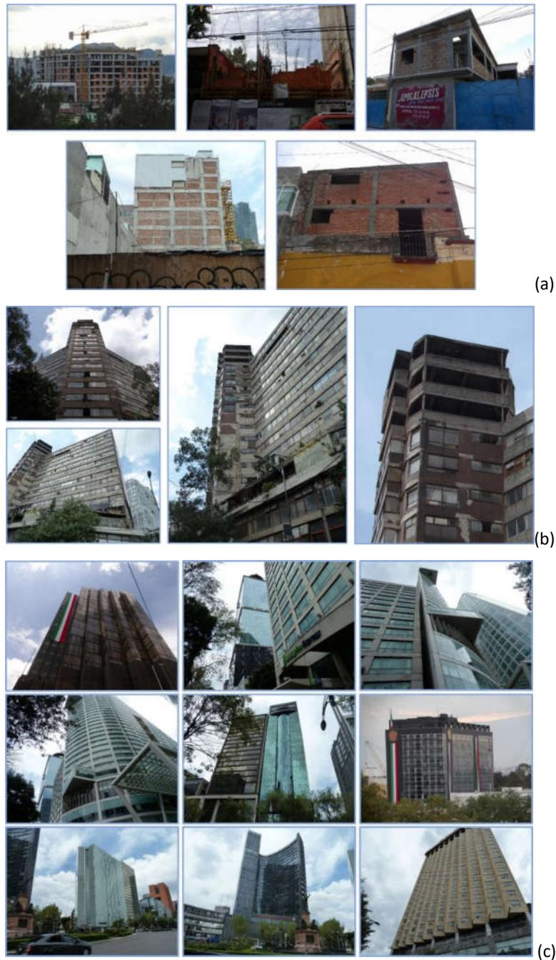
**Figure 5:** (a) Reinforced-concrete buildings with non-ductile detailing with unreinforced infill walls comprising bricks, clay tiles or concrete blocks with bricks being the most common material. (b) Pre-1985 high-rise reinforced concrete buildings in Mexico City with unreinforced brick infill walls. (c) Modern high-rise reinforced concrete buildings in Mexico City with unreinforced brick infill walls (from Lekkas et al. 2017).
