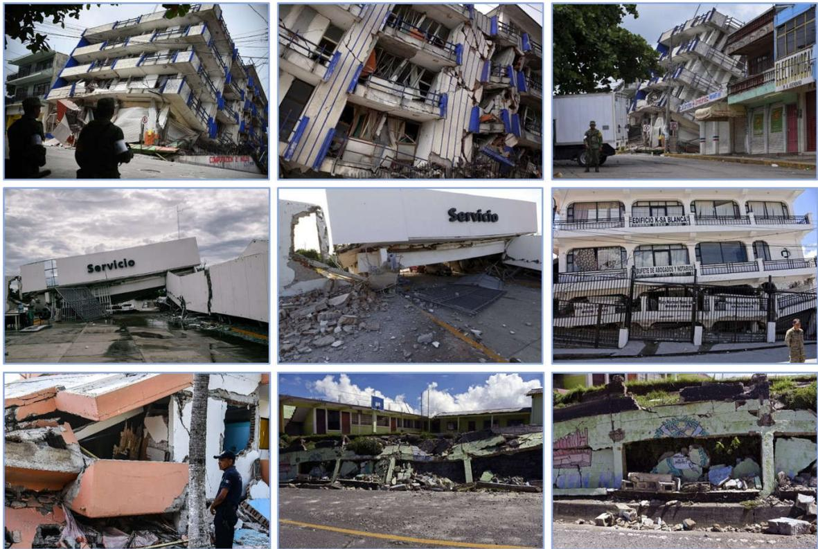
Figure 12: R/C buildings in Oaxaca State with damage induced by the September 7, 2017 earthquake.
