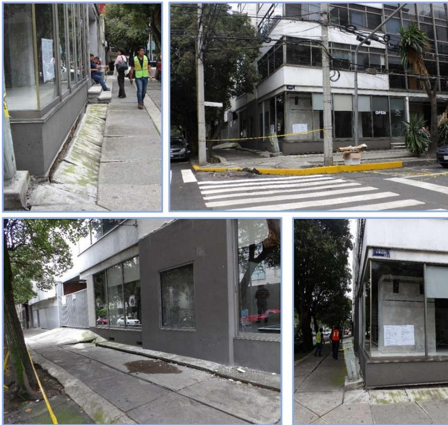
**Figure 15:** Tilting of buildings in Mexico City due to the September 19, 2017 earthquake and the related differential displacement affecting the building foundation (from Lekkas et al. 2017). The structural components of the building were generally undamaged.
