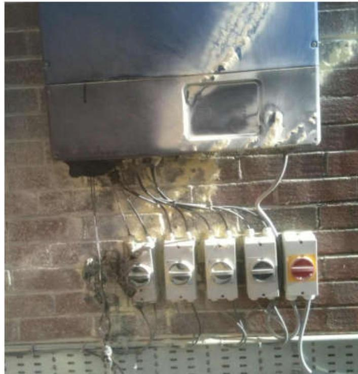
Figure 8. Localized PV fire where the left DC isolator is completely missing with the next DC isolator and inverted also being damaged by fire (BRE 2017)
