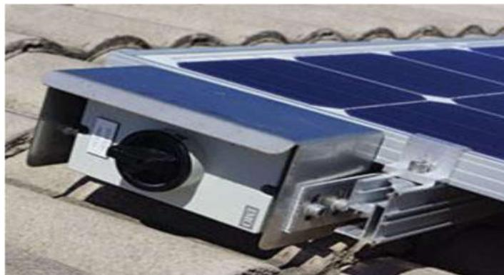
Figure 4: Solar PV system with a rooftop installed DC isolator switch (Chiaromonte et al 2016)
