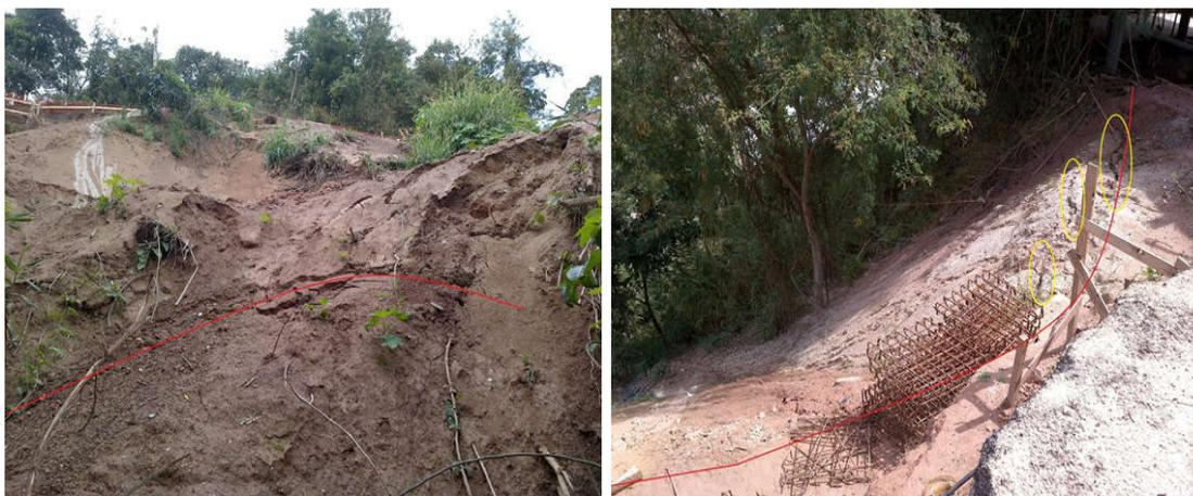
Image 02 - Soil of colluvium deposited in the base and the face of the slope in past events
