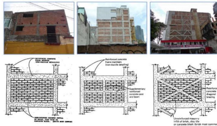
**Figure 6:** Typical methods for reinforcing masonry infill: diagonal cross-bracing frequently used in low-and medium-rise constructions.
