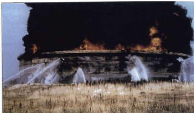
Figure 3. External cooling of tank walls in a full surface fire (HM Fire Service Inspectorate 2000)
