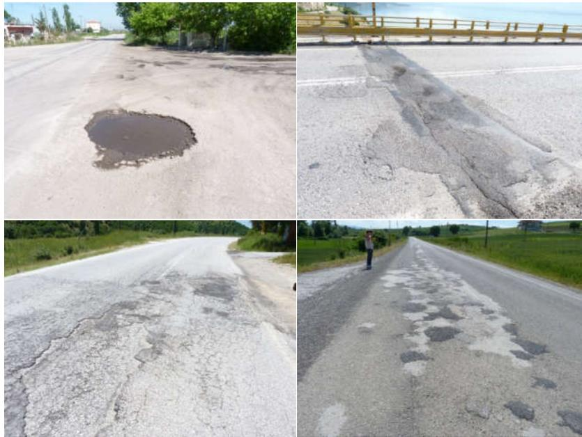
**Image 6:** Examples of poor road maintenance as a cause of increased rate of accidents in the Region of Western Macedonia (Karadimou M. et al, 2012)
