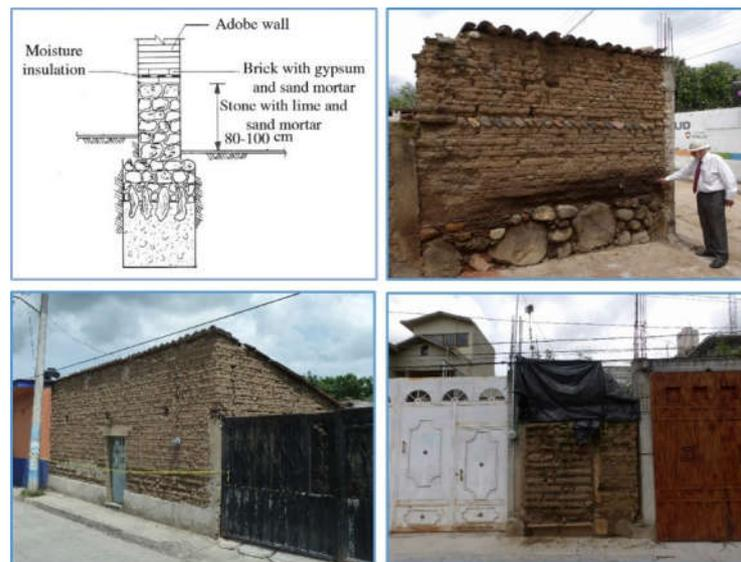
**Figure 8:** Details of the foundations of the adobe buildings (up left) and details of adobe structures that comprise the majority of buildings in Pueblas and Morelos states of Central Mexico.
