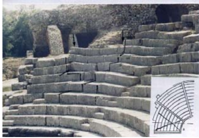
Figure 1. Photograph of the Butrinti Amphitheatre of the 3 rd century BC. Deformed construction and especially open fissures are shown by arrows at the western side of the auditorium. Right down corner: the sketch of the diagonal shear cracks. They are typical evidence of seismic activity.
