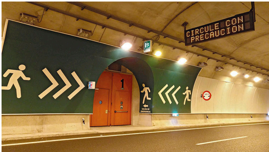
Figure 3. Inside of a tunnel outside of Greece (Source: revistaitransporte.com)
