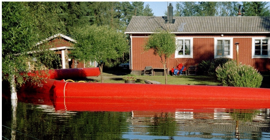
Figure 2. A Tubewall saving a private home in Hälsingland, Sweden, in 2000.
