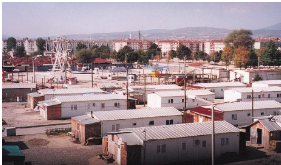
Figure 1: Photo of a transitional settlement in Western Turkey after the 1999 earthquake [2]. The repetition of improvised parts in Prefabricated Units are perceived as an improvisation trend that solves a problem or meets a spatial need. Following the prevalence of these practices, a trend emerges in the local market for specific materials or technical knowledge.
